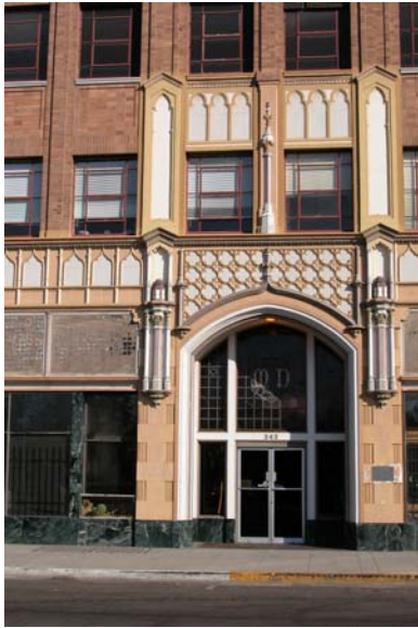
Well-defined entrance to a Stockton building.
