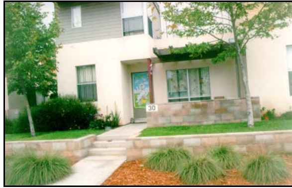
Low retaining walls in the front yard
