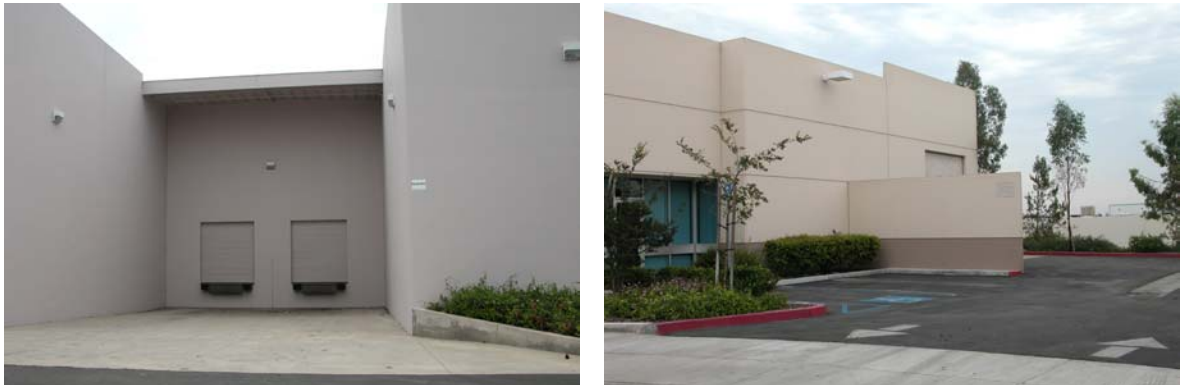
Recess loading docks into buildings and use wing-walls to screen loading areas.
