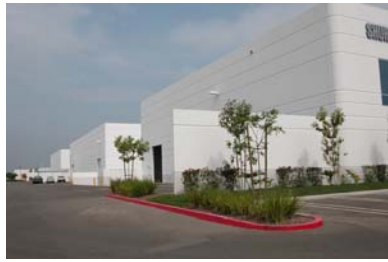
Landscaping and wing-wall screen loading area.
