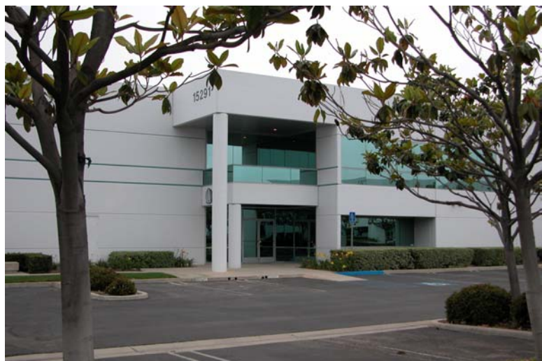
The building's entry should be defined by a strong architectural statement.
