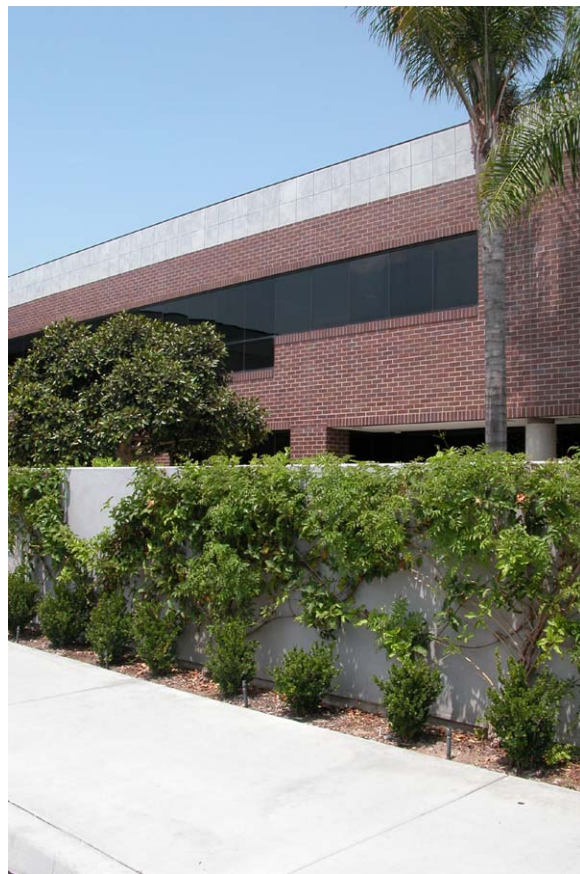
Use vines on walls to deter graffiti.
