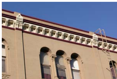
Example of restored cornice detail.
