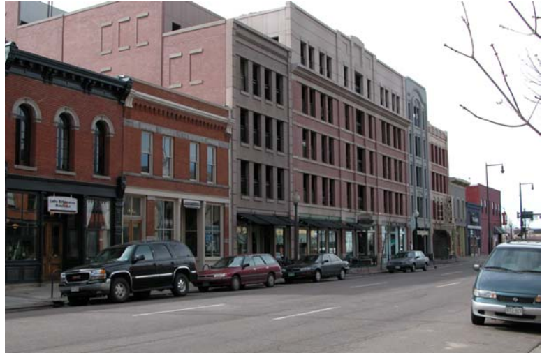
This parking garage fits well with adjacent buildings by maintaining openings of similar size and proportion.
